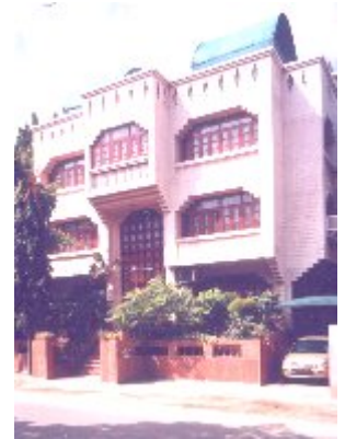
SAI (H.O. Building, Ahmedabad)
